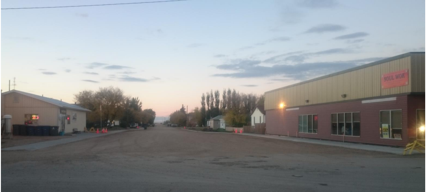
4 th street road work, new sidewalks and curbs.
